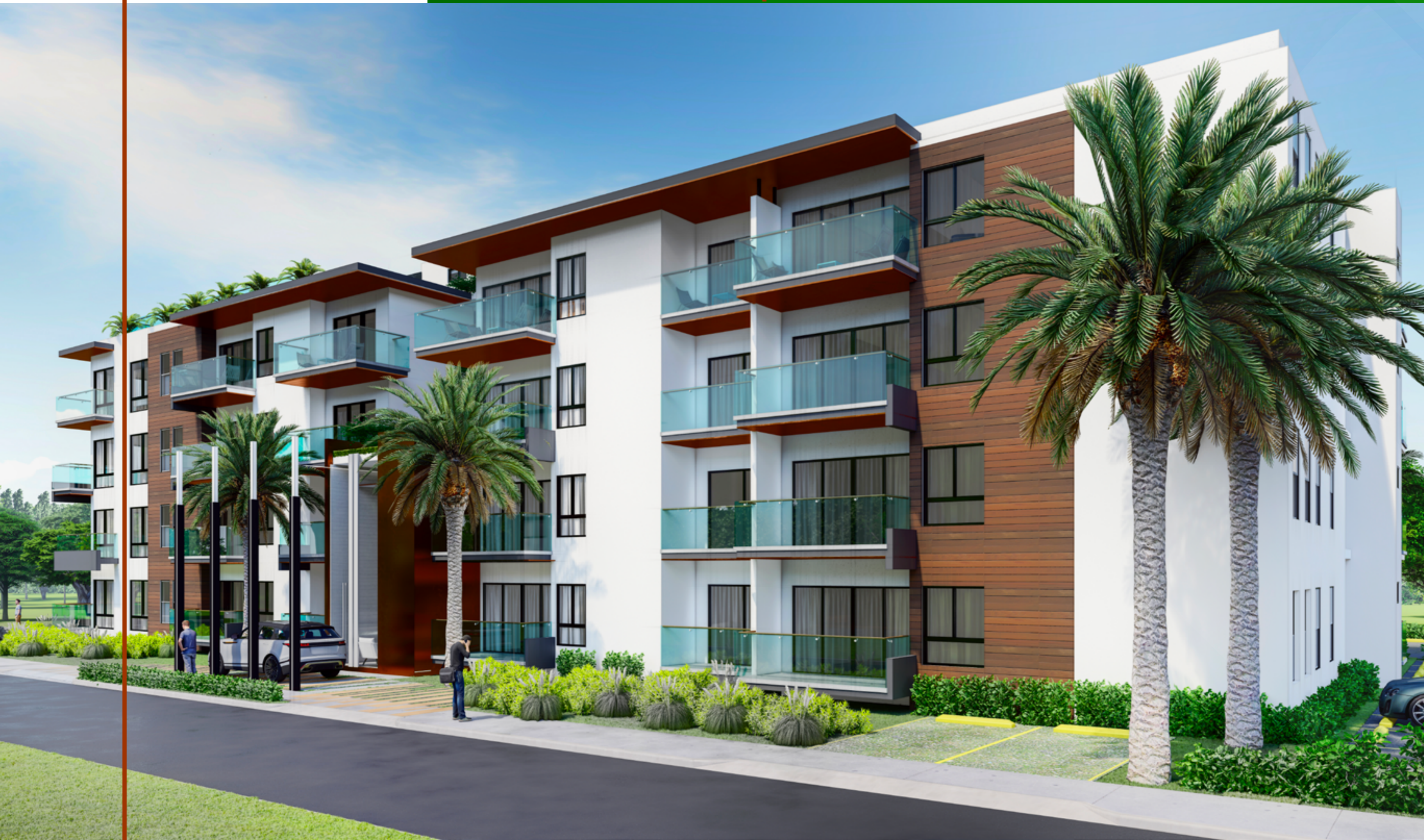
Parkwest exterior view
